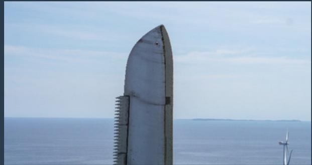
In late 2017 Cyberhawk was tasked by Siemens Gamesa to carry out visual inspections of 27 wind turbines at an offshore wind farm<sup>[3]</sup>. Unique to this inspection campaign was the requirement to develop a bespoke app to meet specified requirements: a 25% overlap in images to ensure no blade surface was missed. In this case the images of each individual turbine were processed and uploaded on the same day as inspection.
